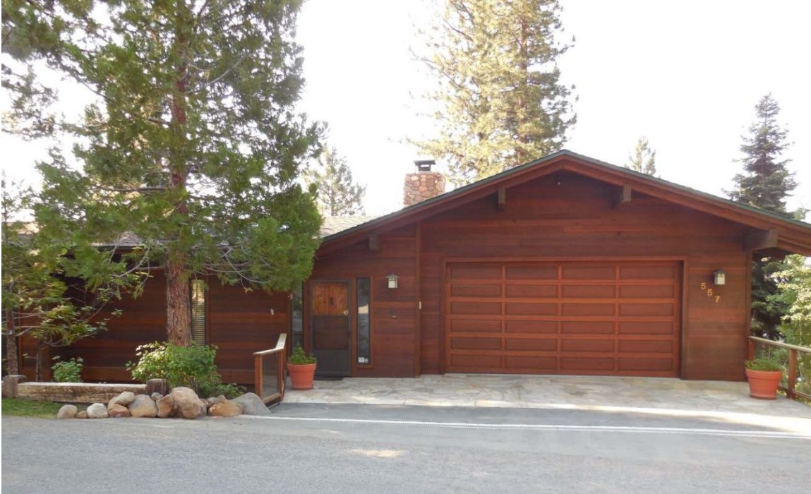
557 Dale Drive (Subject property). The front door on the left extending two feet beyond the garage face.
